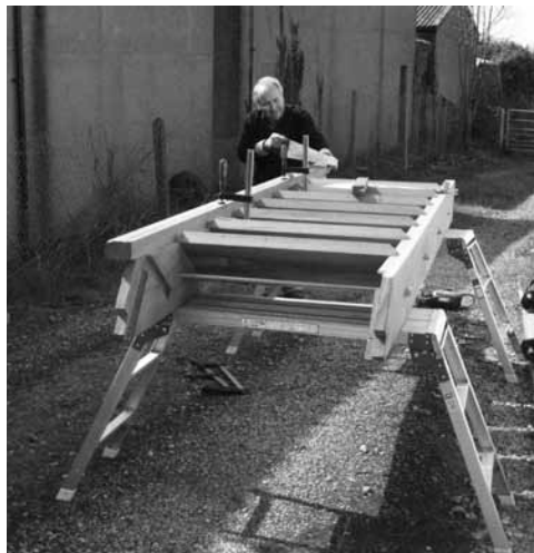
Constructing the steps
